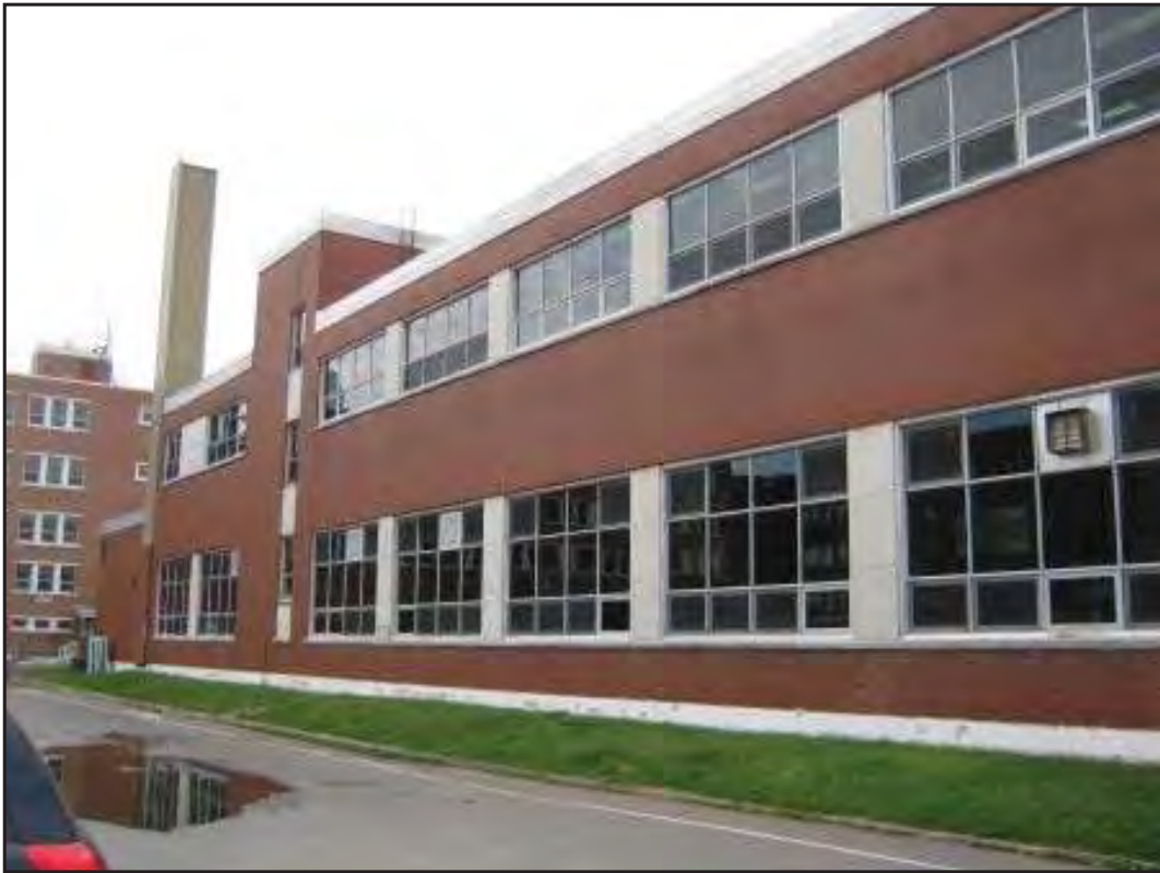
The western adjoining property. Photo looking south.
