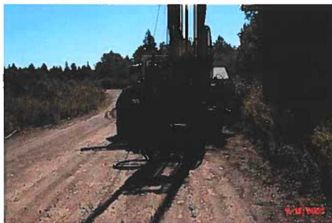
Photo 11 – Saddle Dyke 2 – Probe hole on crest
