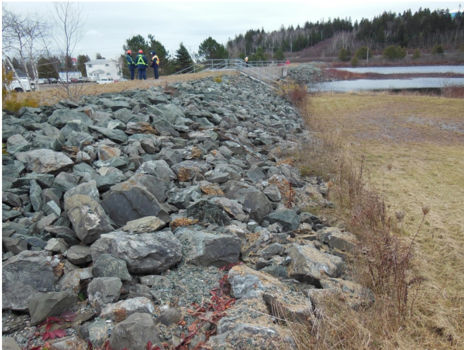
Photo 33: Spruce Lake Dam – Left Embankment Upstream riprap protection
