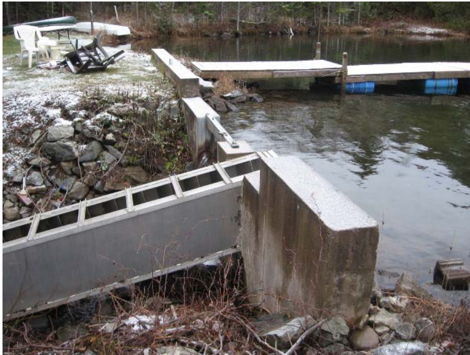
Photo 44: Hunter Lake Dam Downstream face of the dam
