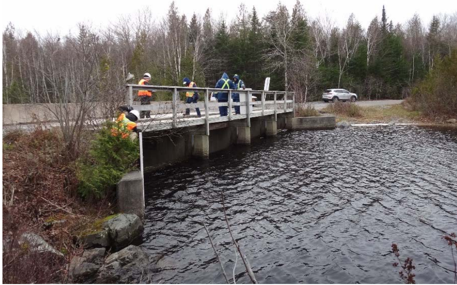
Photo 1: Menzies Lake Control Structure View from upstream of left abutment
