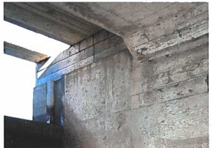
Photo 6 – Bay 2 – Underside of stoplog deck.
