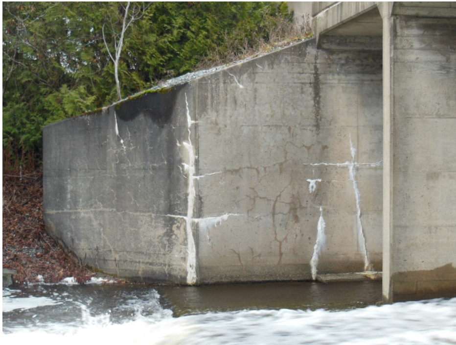
Photo 9: Menzies Lake Control Structure Right downstream wingwall
