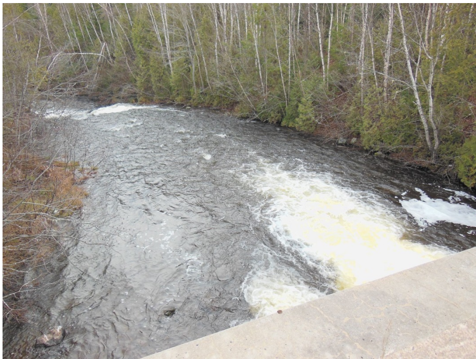
Photo 4: Menzies Lake Control Structure Looking downstream from the structure
