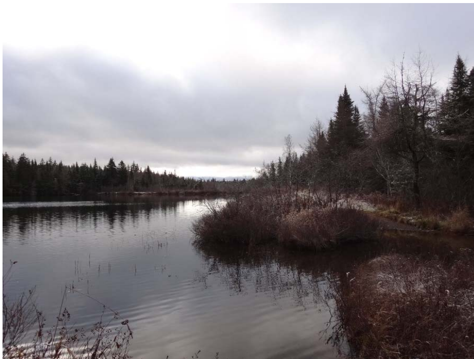
Photo 47: McBrien Southwest Dam View from beyond the breach at right abutment
