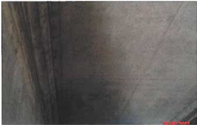
Photo 13 – Underside of concrete deck
