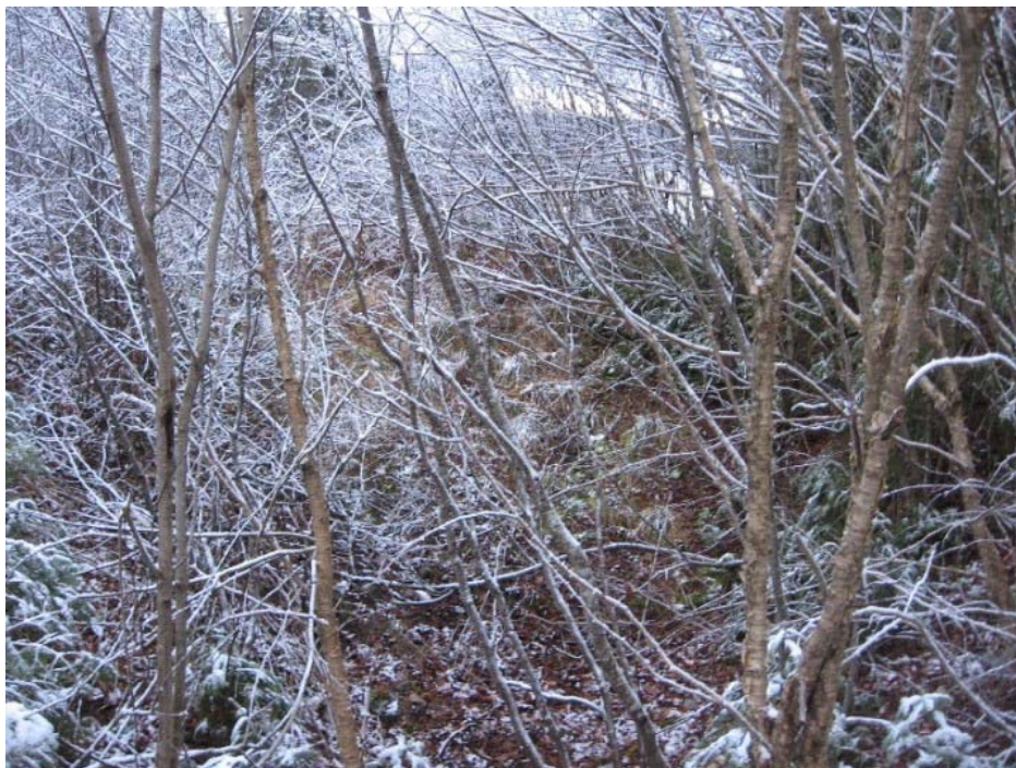
Photo 63: Taylor Lake Dam Looking towards downstream face of dam
