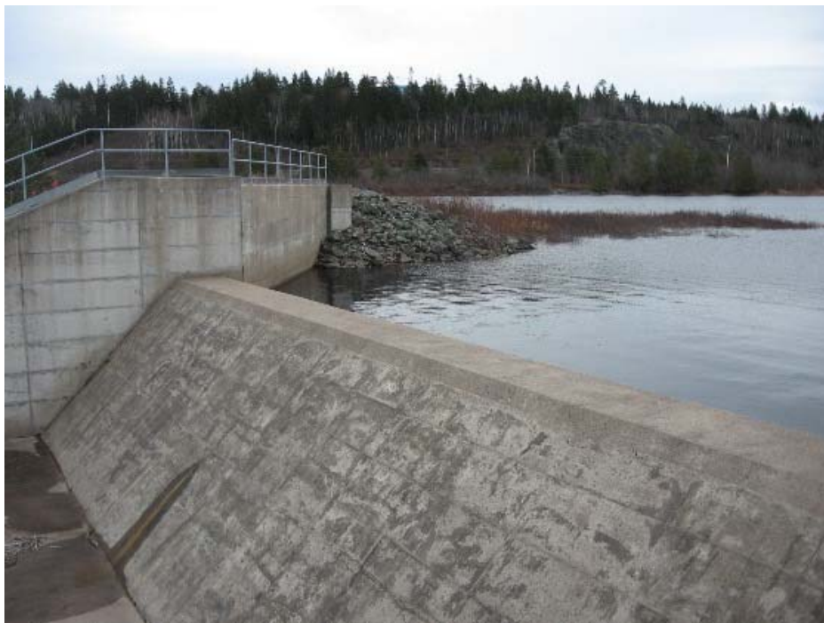
Photo 26: Spruce Lake Dam – Concrete Spillway View of downstream slope and crest
