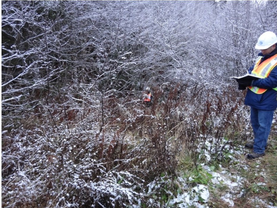
Photo 60: Taylor Lake Dam Looking at crest towards downstream slope (person at toe visible)
