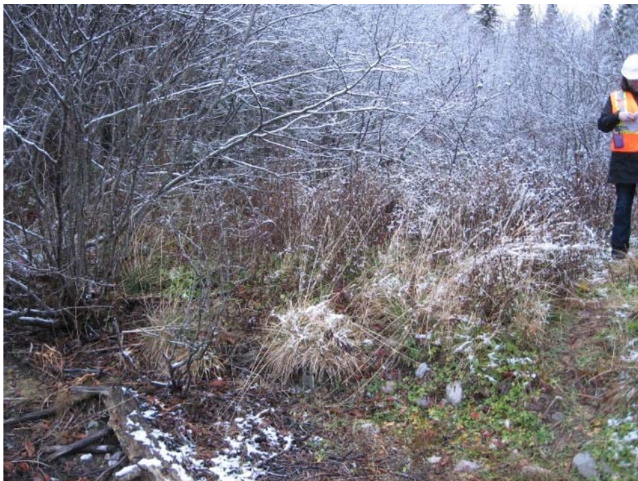
Photo 61: Taylor Lake Dam Upstream slope
