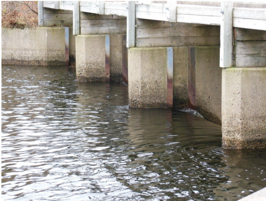
Photo 5: Menzies Lake Control Structure Upstream piers
