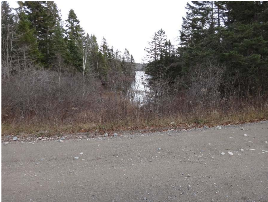
Photo 19: Menzies Lake Saddle Dyke 3 View from crest looking upstream
