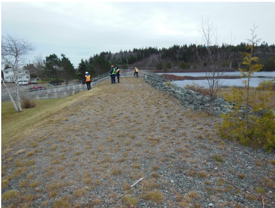
Photo 32: Spruce Lake Dam – Left Embankment View from left abutment
