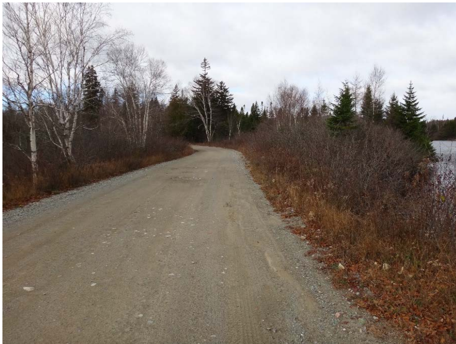
Photo 16: Menzies Lake Saddle Dyke 2 View from left abutment looking West
