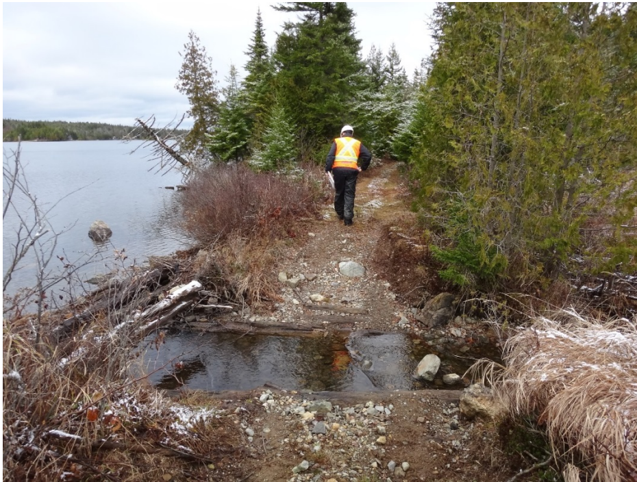
Photo 56: Terreo Lake Dam Crest looking towards left abutment, note breached area and beaverdam upstream
