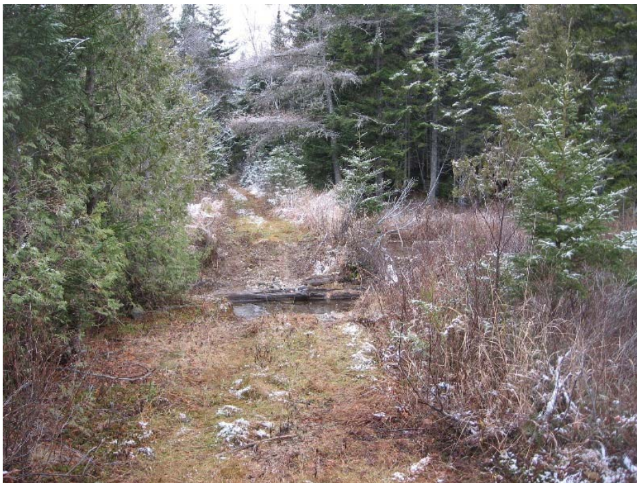
Photo 57: Terreo Lake Dam Crest looking towards right abutment
