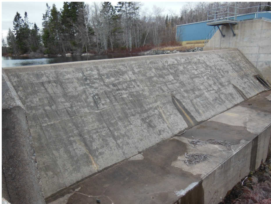
Photo 24: Spruce Lake Dam – Concrete Spillway Downstream face of spillway
