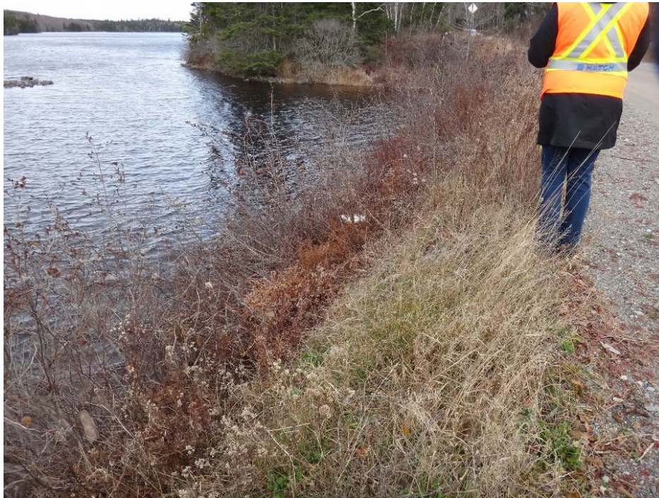
Photo 15: Menzies Lake Saddle Dyke1 Upstream slope
