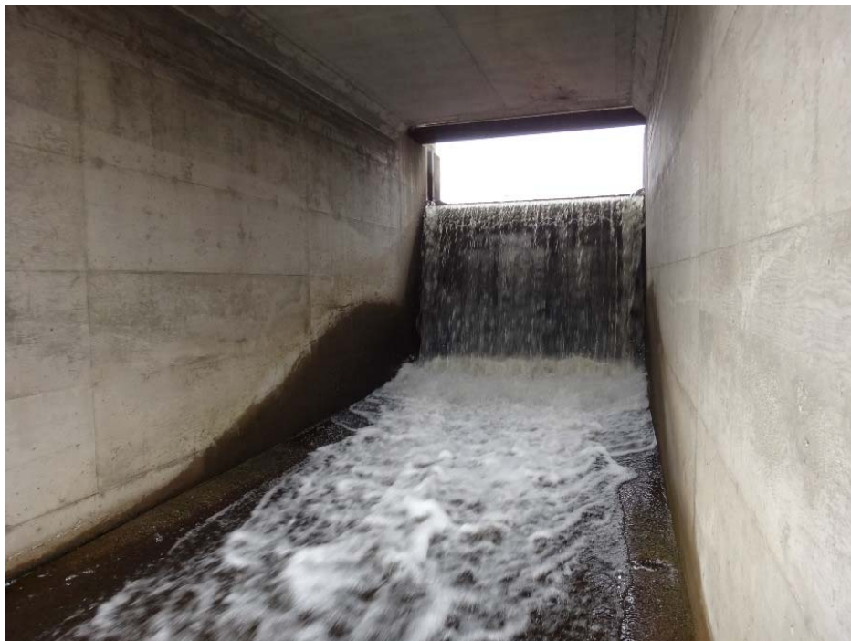
Photo 12: Menzies Lake Control Structure Flow over stoplogs
