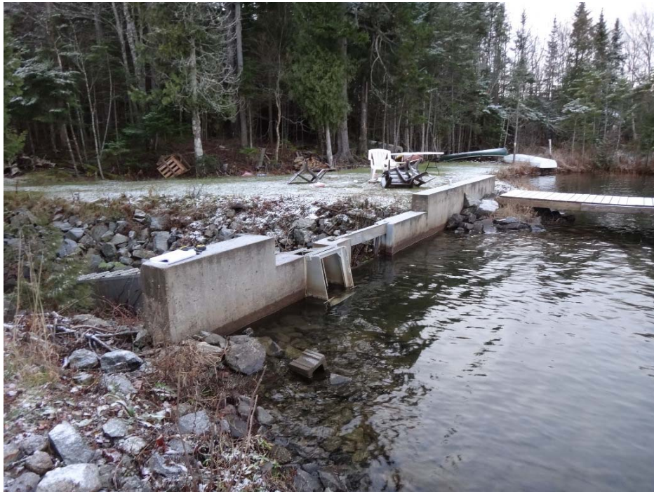
Photo 42: Hunter Lake Dam View of upstream face of structure
