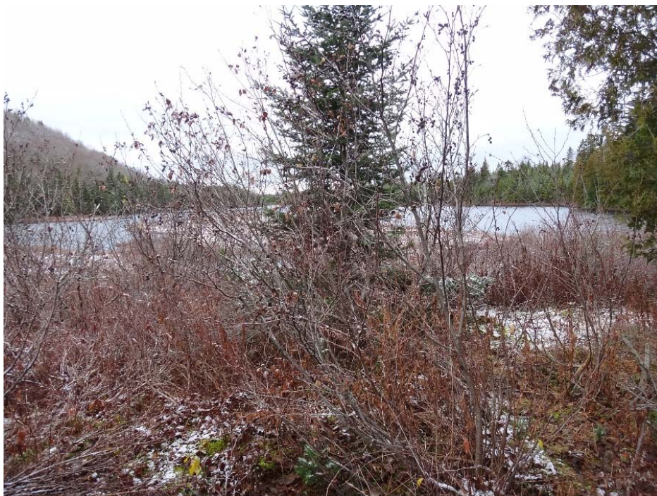
Photo 55: McBrien Southeast Dam Looking upstream
