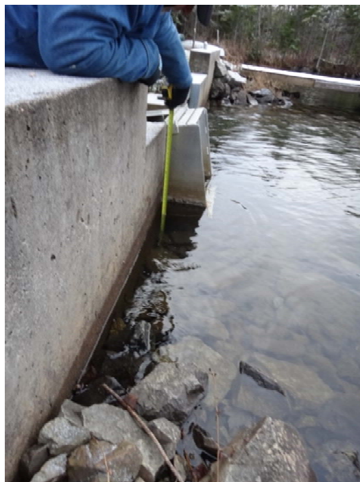
Photo 43: Hunter Lake Dam Sedimentation in reservoir upstream of the dam
