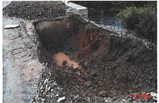
Photo 16 – Test pit in right abutment
