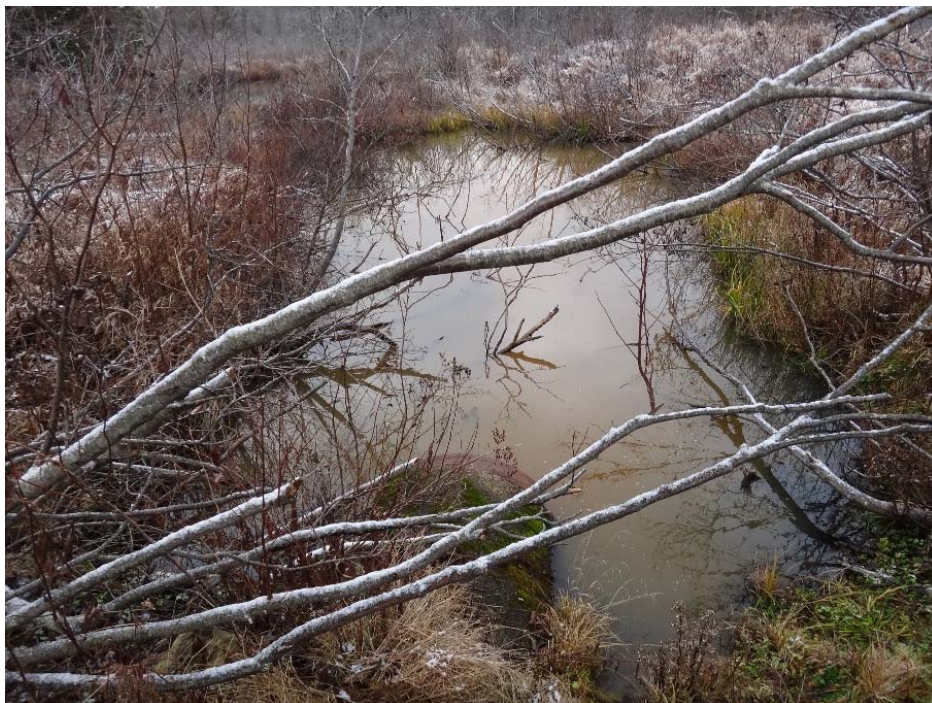
Photo 51: McBrien Southwest Dam
