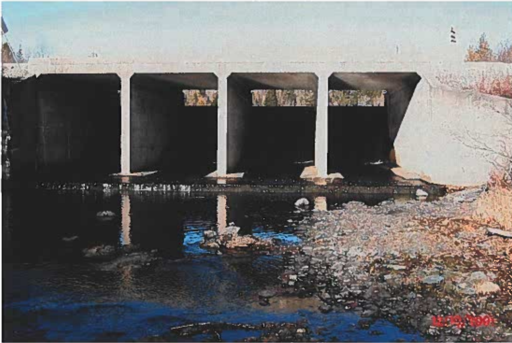
Menzies Lake Control Structure Looking from Downstream
