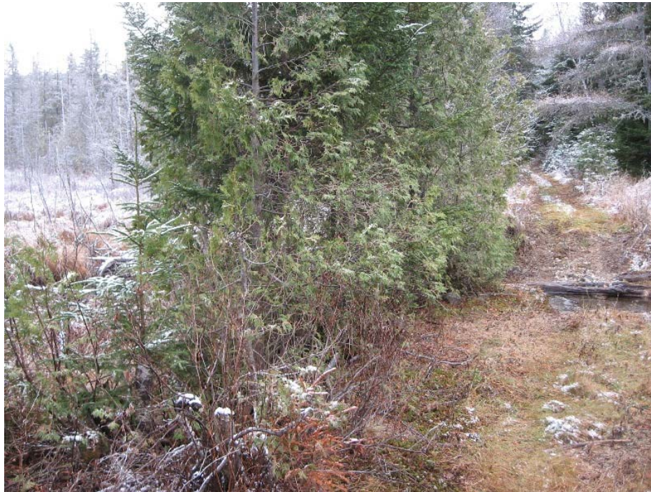
Photo 58: Terreo Lake Dam Crest and downstream slope
