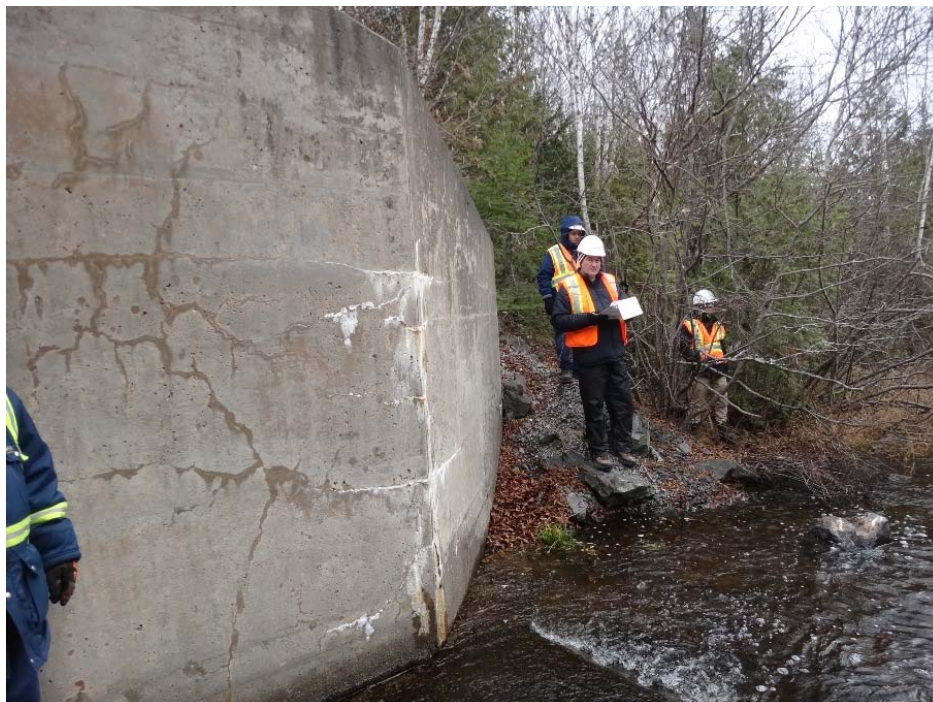
Photo 8: Menzies Lake Control Structure Left downstream wingwall
