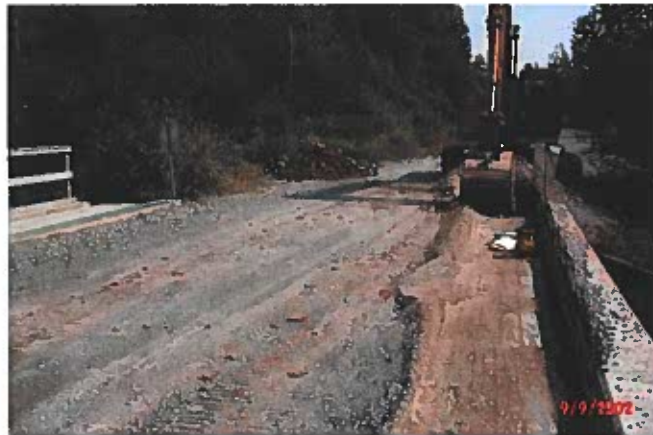
Photo 17 – Deck and test pit in left abutment
