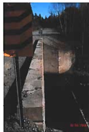
Photo 12 – Left downstream wingwall
