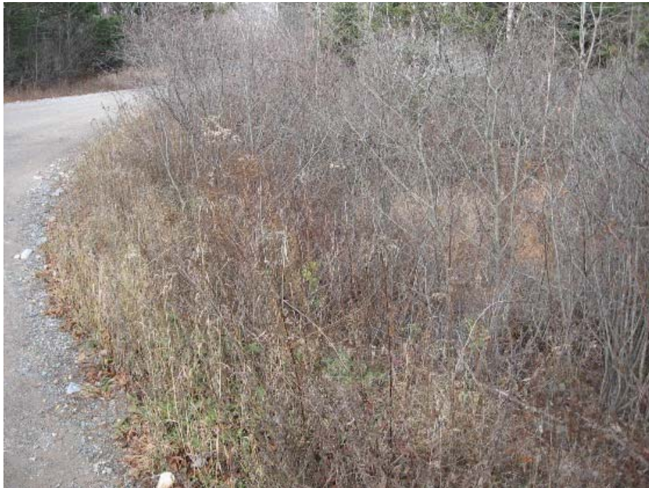
Photo 21: Menzies Lake Saddle Dyke 3 Upstream slope
