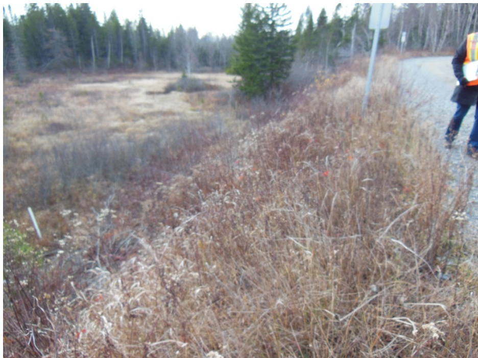
Photo 14: Menzies Lake Saddle Dyke 1 Downstream slope and wetland type area downstream.
