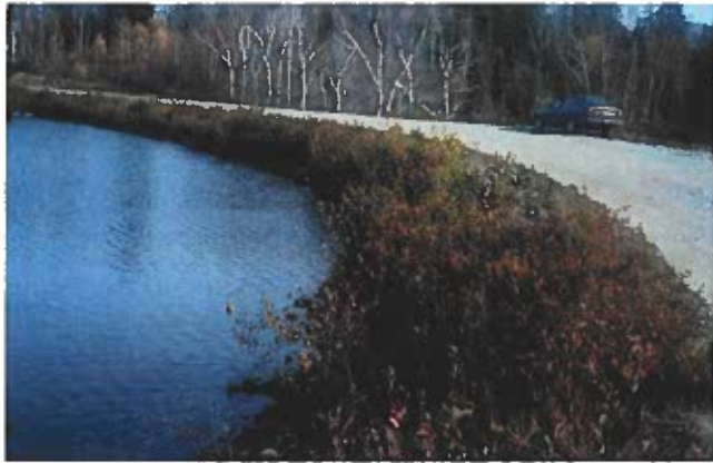
Photo 1 – Saddle Dyke 1 from Upstream Right
