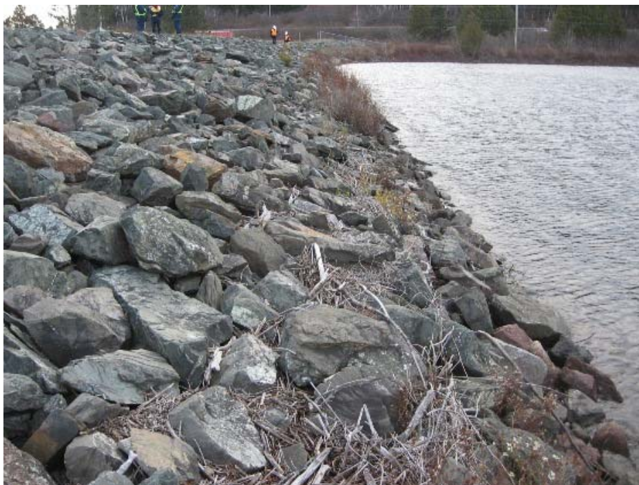
Photo 38: Spruce Lake Dam – Right Embankment Upstream riprap protection and driftwood debris
