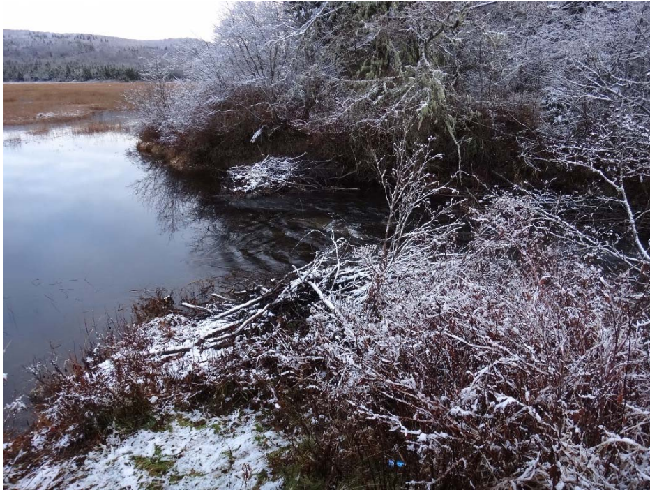
Photo 64: Otter Lake Dam Breach at Otter Lake Dam
