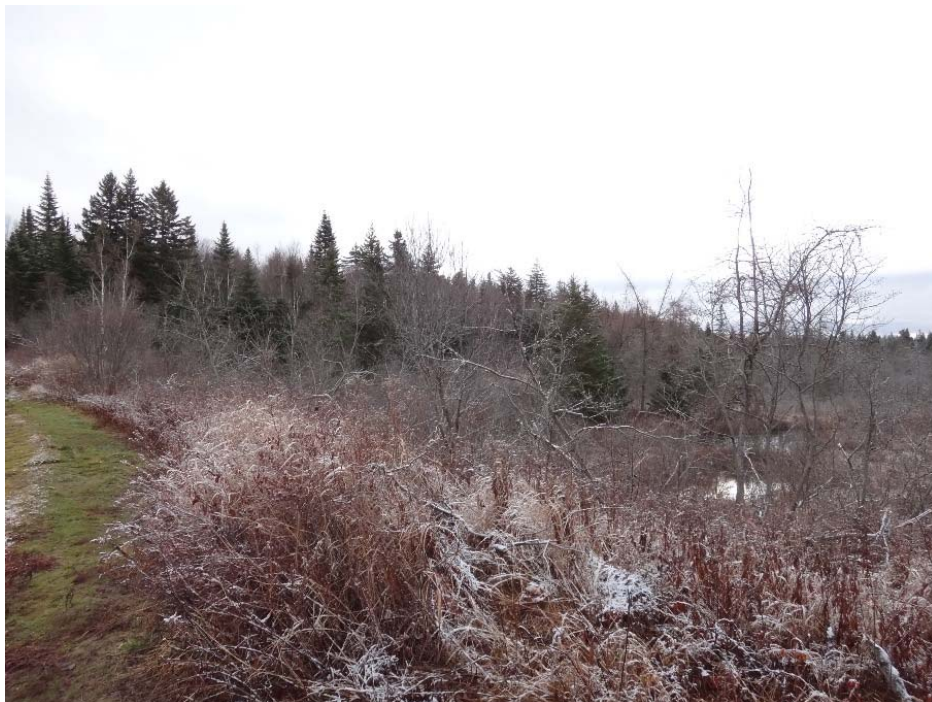
Photo 53: McBrien Southwest Dam
