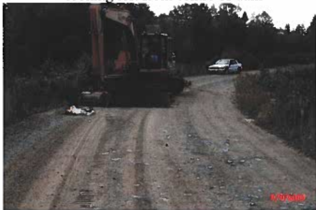
Photo 9 – Saddle Dyke 1 – Test pit on crest
