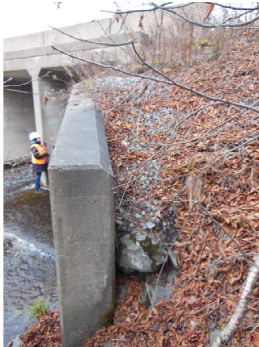
Photo 7: Menzies Lake Control Structure Left downstream wingwall
