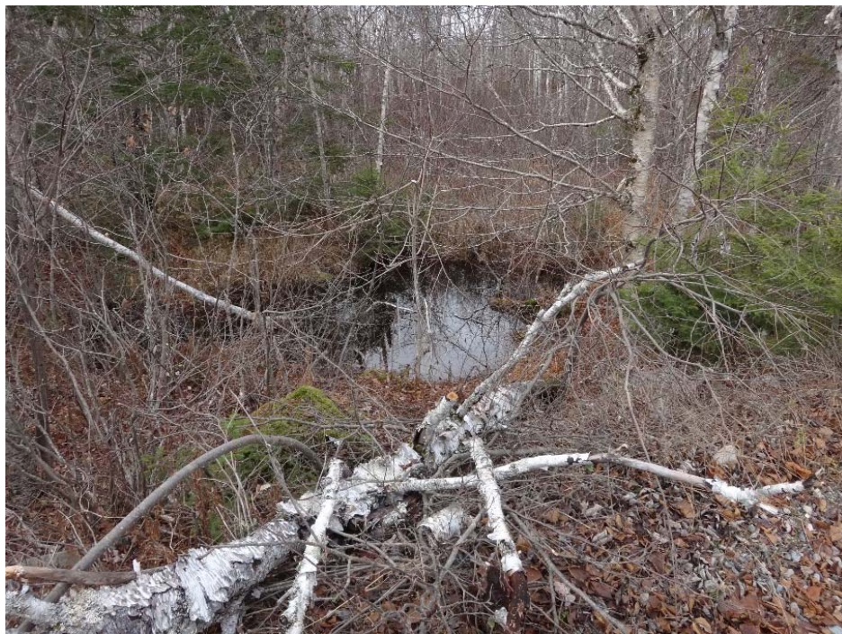
Photo 22: Menzies Lake Saddle Dyke 3 Downstream slope and ponded water downstream
