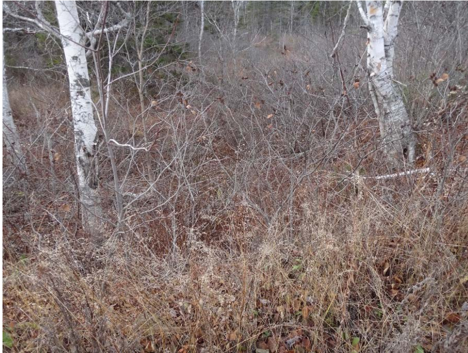
Photo 17: Menzies Lake Saddle Dyke 2 Trees and brush on downstream slope
