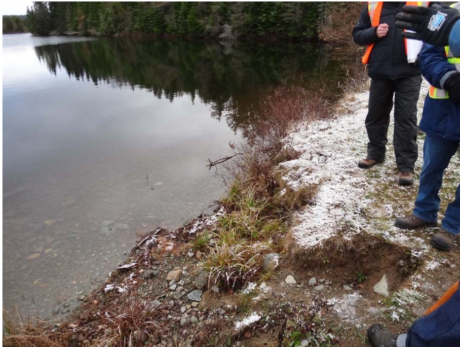
Photo 52: McBrien Southwest Dam
