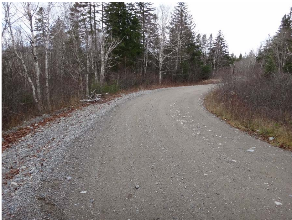
Photo 20: Menzies Lake Saddle Dyke 3 At left abutment crest looking North
