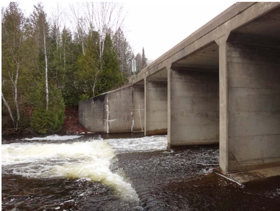
Photo 10: Menzies Lake Control Structure View of structure from downstream left wingwall
