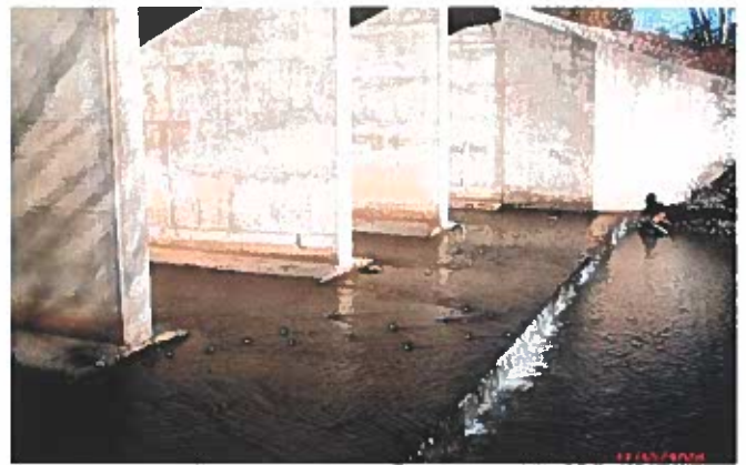
Photo 8 – End of piers and slab extension
