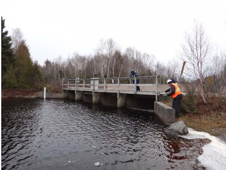
Photo 2: Menzies Lake Control Structure View from upstream of right abutment
