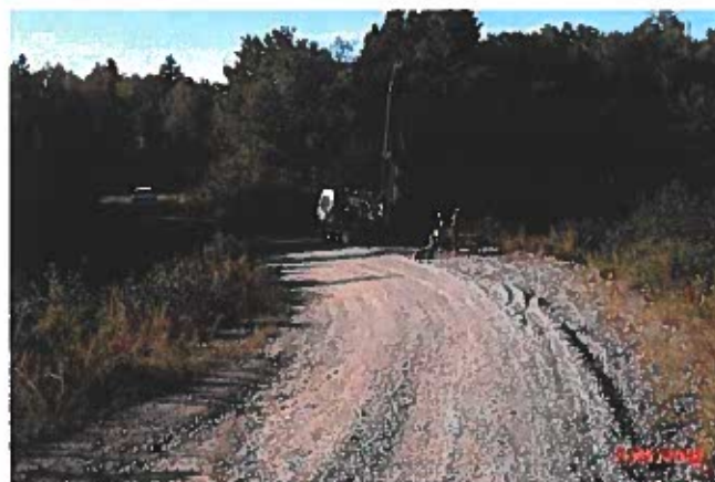
Photo 12 – Saddle Dyke 3 – Probe hole on crest
