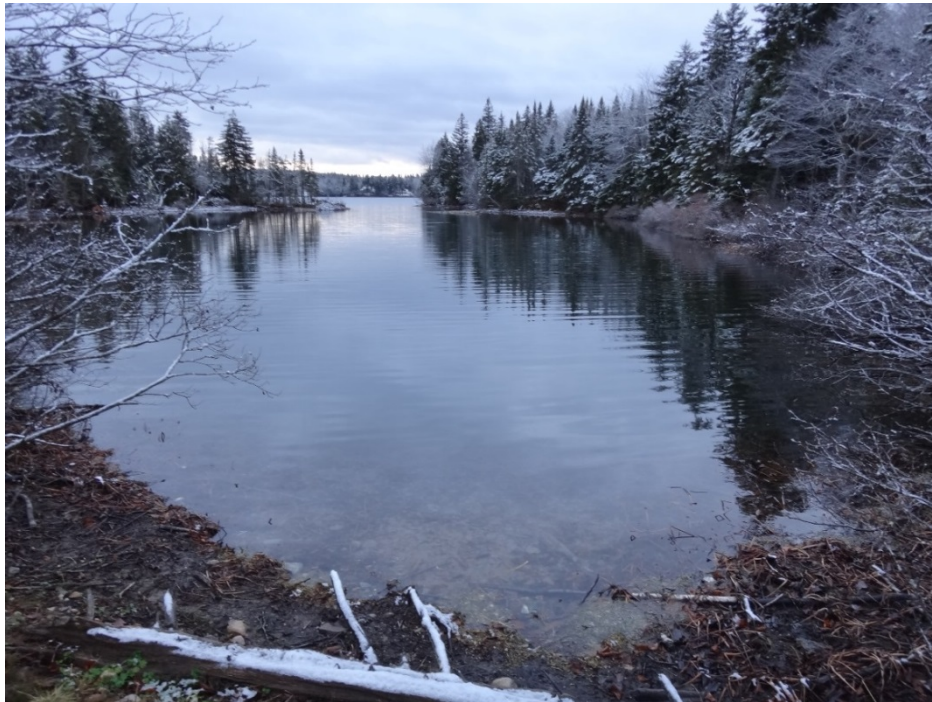
Photo 62: Taylor Lake Dam Looking upstream from dam
