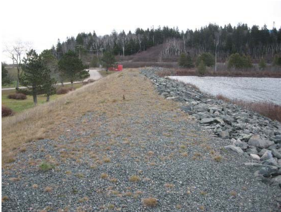
Photo 37: Spruce Lake Dam – Right Embankment View from abutment with spillway
