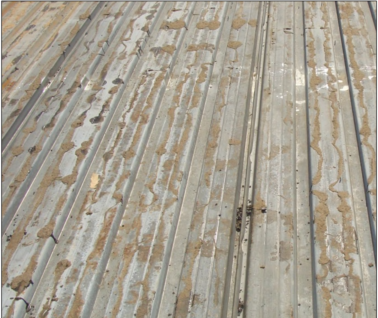
Photo of Level 1: No Visible Corrosion
