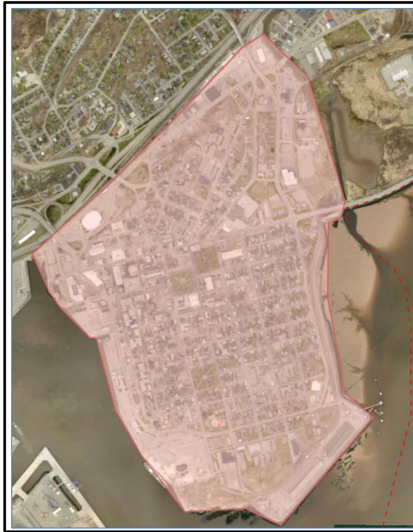
Figure 1: Approximate Central Peninsula Combined Sewer Separation Study Area
