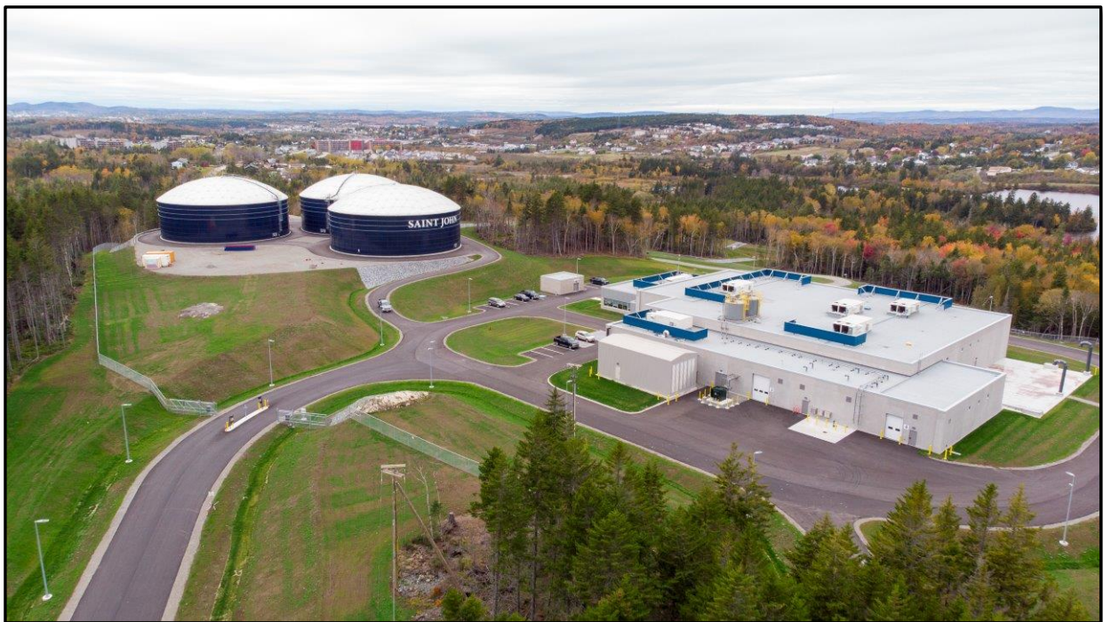
Loch Lomond Drinking Water Treatment Facility September 2018
