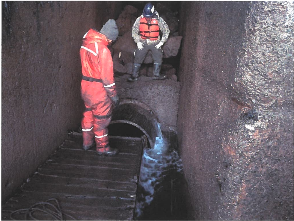
Figure 1: HDPE Sliplining at Outfall - Before Tideflex Install
