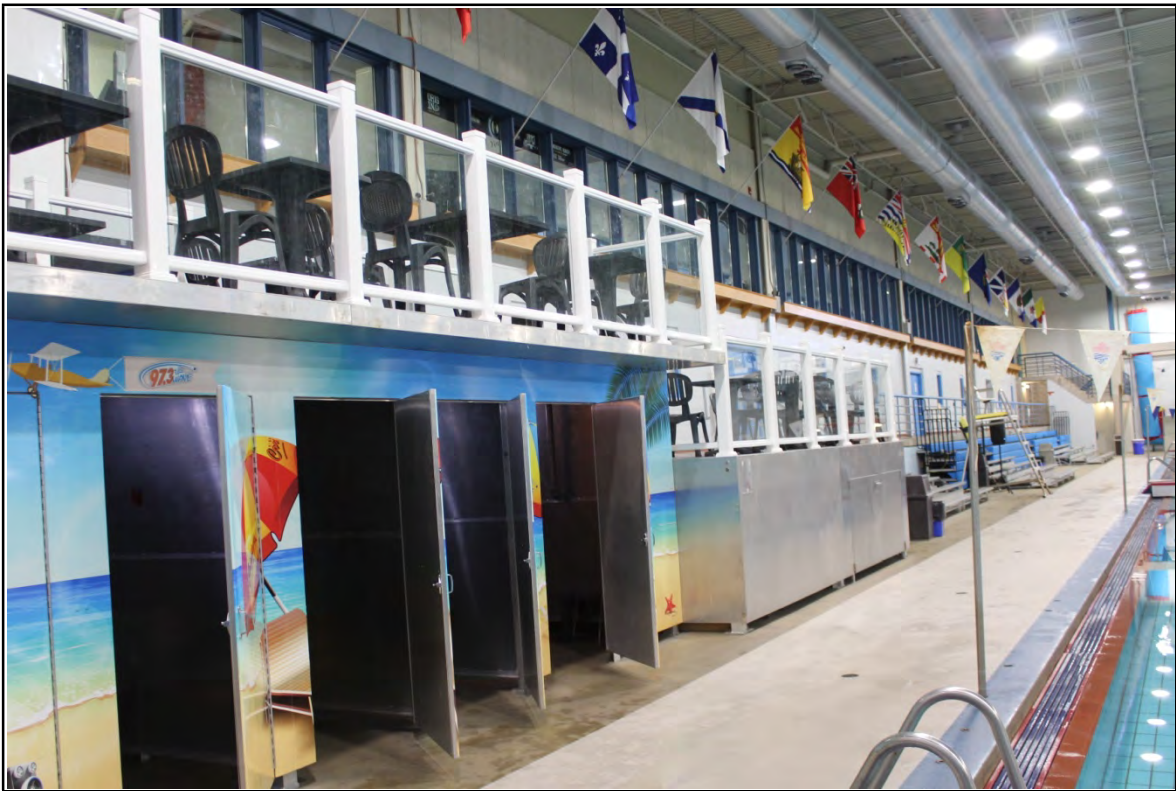
Photo 16: Aluminum Pool Side Change Rooms And Mezzanine
