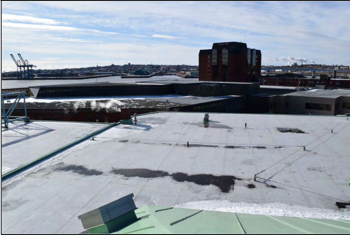
Photo 9: Modified Bitumen Roofing
