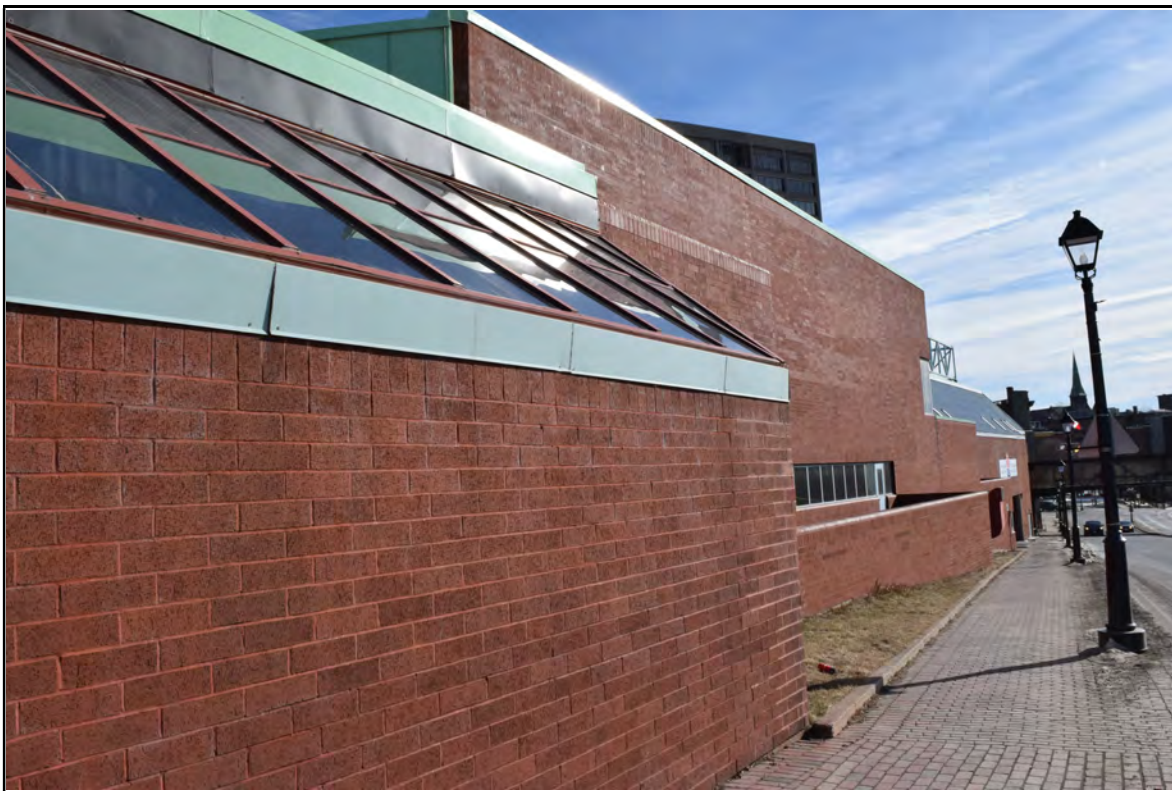
Photo 4: Brick Veneer and Glazing
