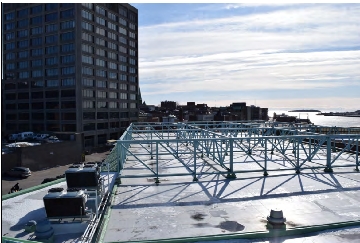
Photo 8: Modified Bitumen Roofing and Metal Frame on Roof
