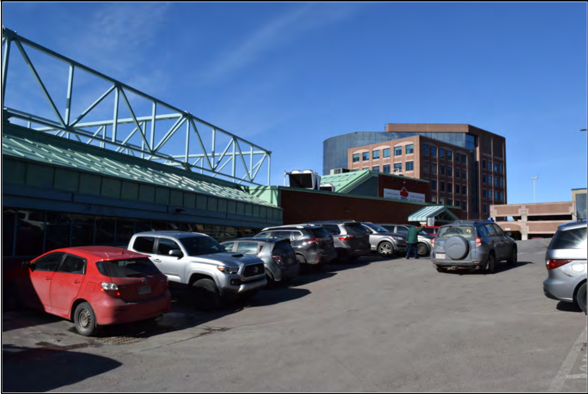
Photo 1: Asphalt Paved Parking Area
