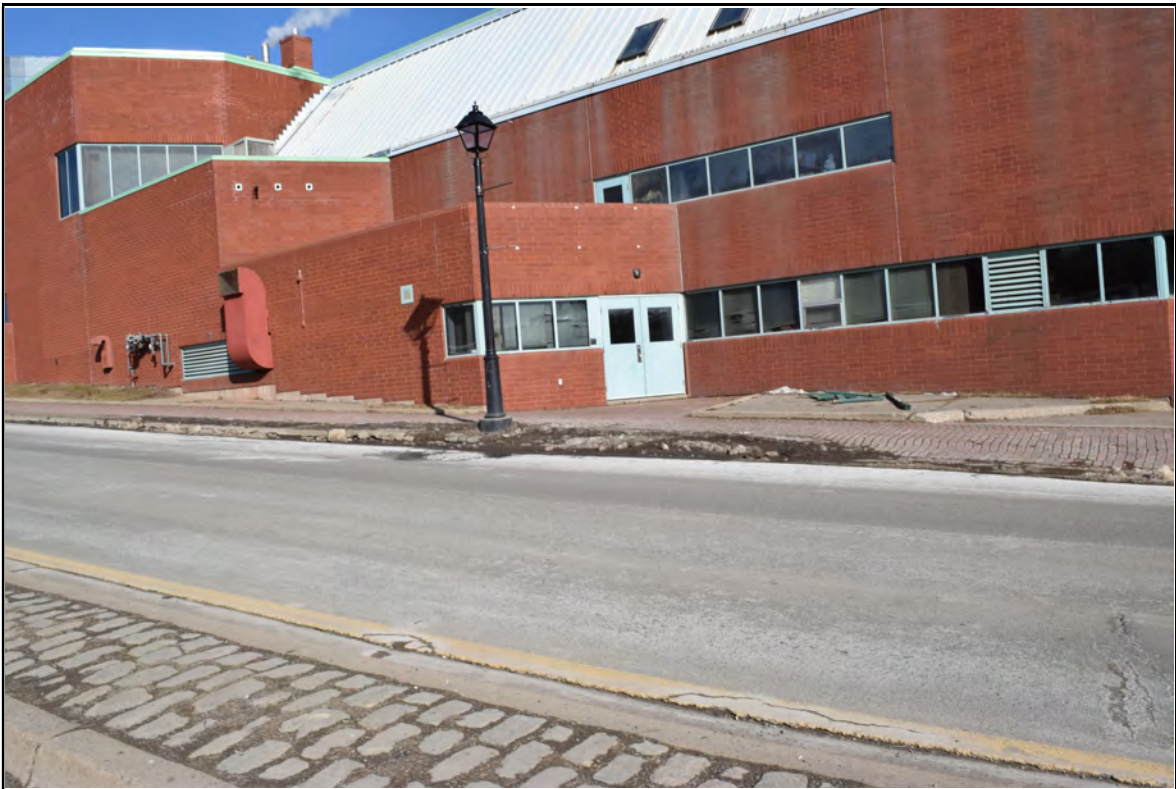
Photo 6: Exterior Cladding and Secondary Entrance Doors
