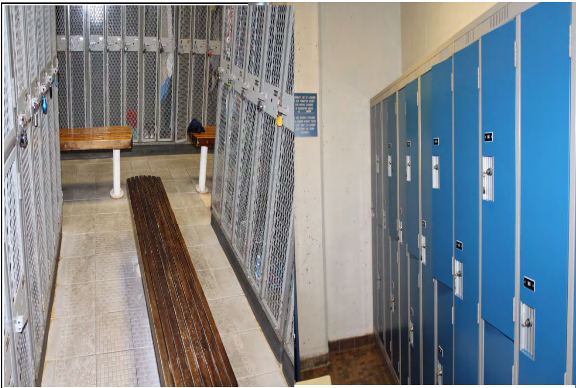
Photo 20: Typical Locker-room Finishes
