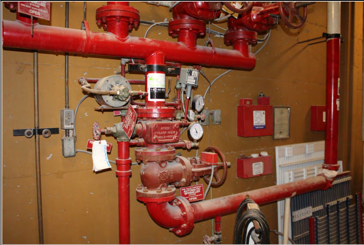
Photo 31: Sprinkler Tree
