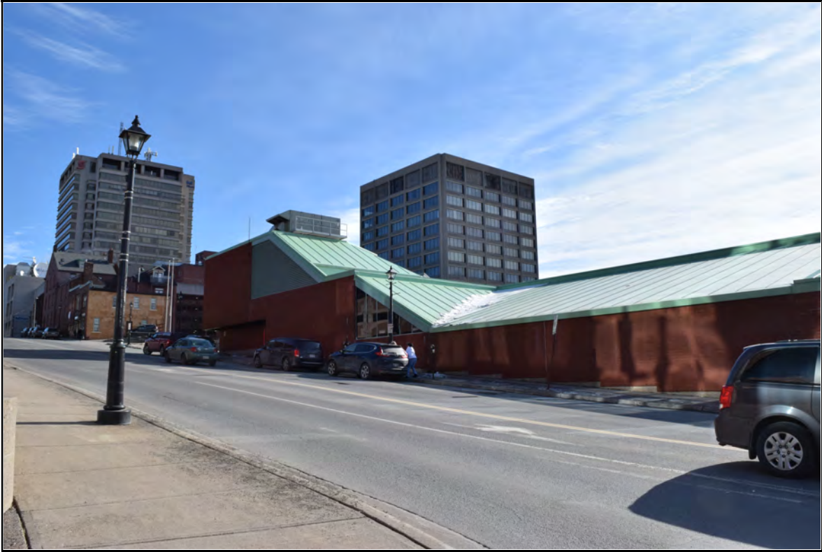
Photo 5: Exterior Brick Veneer and Sloped Metal Roofing
