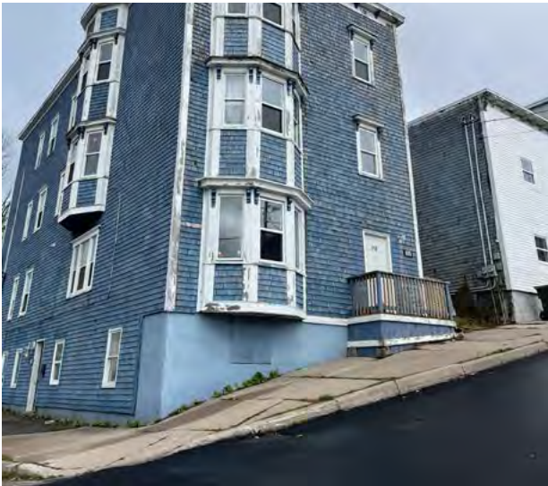
Figure 21: Challenging topography in the planning area. Source: Fotenn
