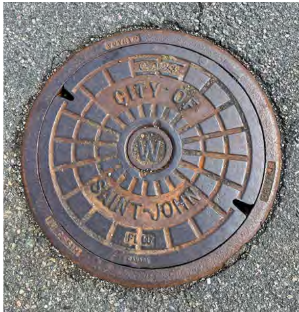
Figure 12: Standard Manhole, Saint John. Source: Fotenn
