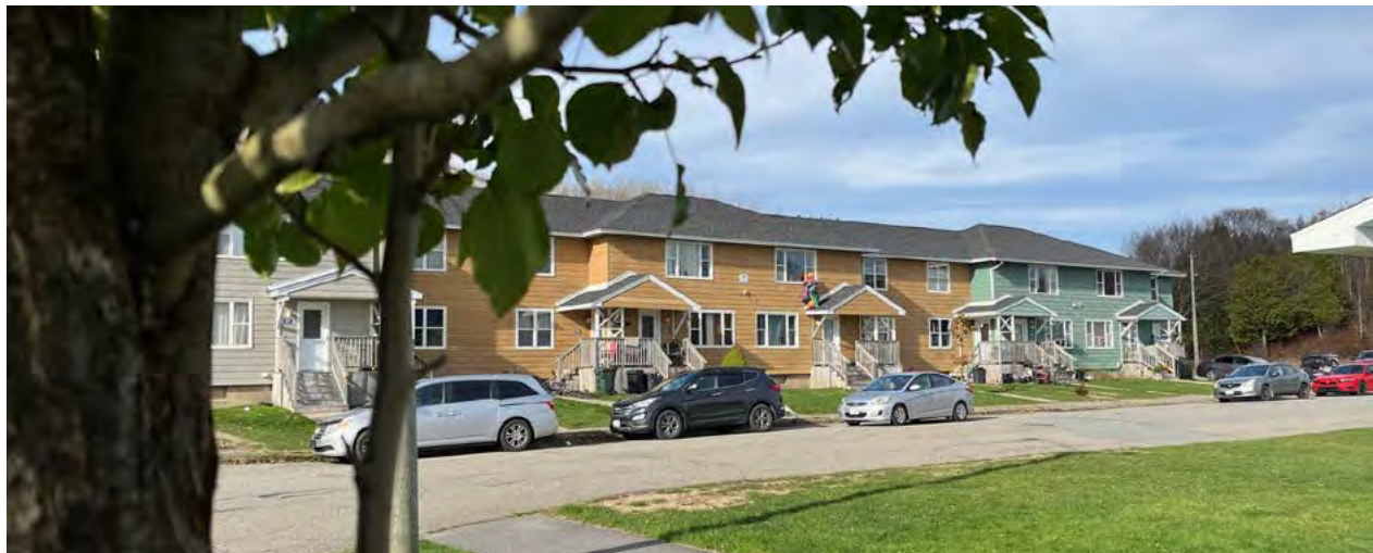
Figure 44: Crescent Valley community, Somerset, Saint John. Source: Fotenn
