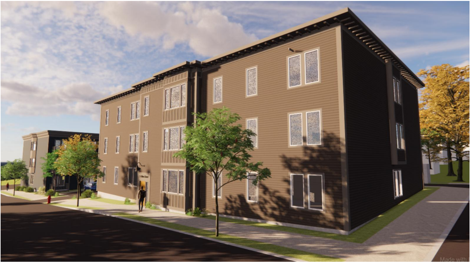
Building 3 – 18 Unit Building Fronting on Albert Street
